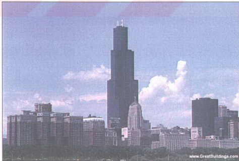
Şekil 2.5 Sears Tower, Chicago, Illinois, 1974-1976 ( www.greatbuildings.com)[3]
