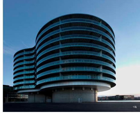
Home Back to last page Previous project Next project Website Frosilos 129 Frosilos Copenhagen, Denmark Realised 2005
