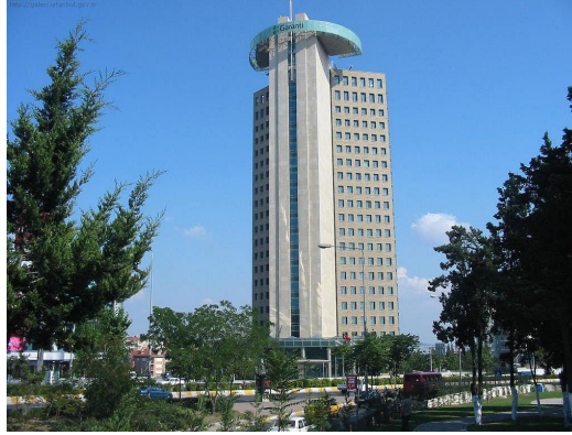
Şekil 5.44 Garanti Bank Headquarters [133]
