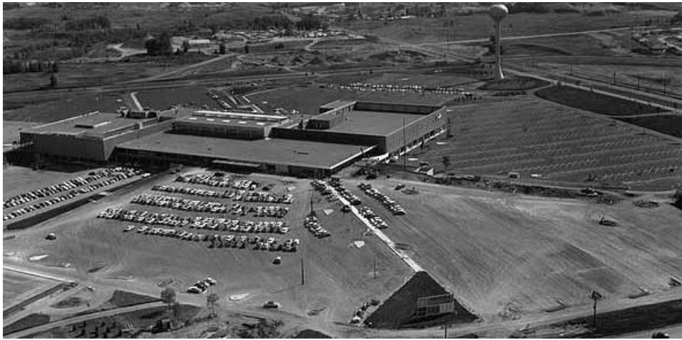
Şekil 2.9 Southdale Center, Minneapolis (history.sandiego.edu, 2009)
