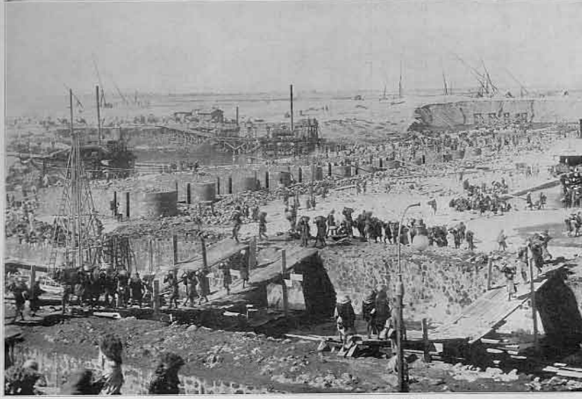
VIEW FROM THE WEST LOCK WALL, SHOWING THE UP-STREAM SIDE OF THE PIERS.
