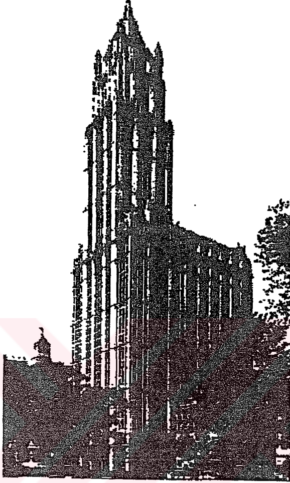
Şekil 1.1 Woolworth Tower Binası New York 1913 (Tall, 1964)
