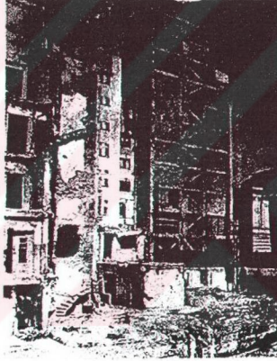
Fig. 32 Foundations of totally collapsed Bar Continental complex.
